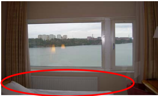
Figure 5.1.8. Example of heat emitter in a typical guest bedroom (Source: Houlihan, 2007)
