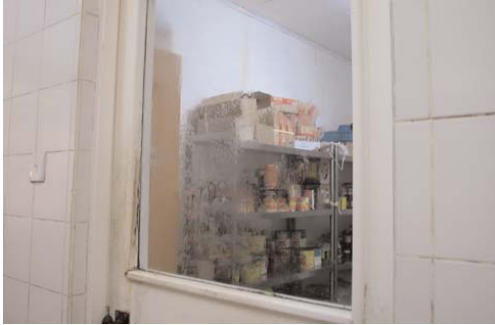
Figure 5.2.3 Condensation on cold store door (XCO2, 2006).
