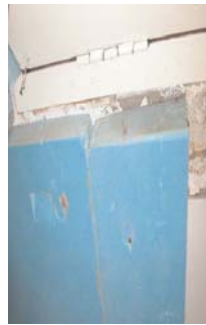
Figure 5.2.4 Patchwork insulation (XCO2, 2006).
