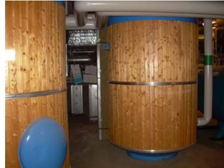
Figure 5.1.9 Hot water storage tanks located in the heating plant room. (photo: Houlihan, 2007)
