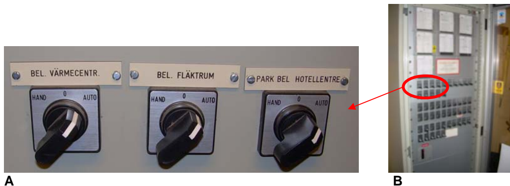
Figure 5.1.12 A and B Zoned heating control panels ( photo: Houlihan, 2007 ).
