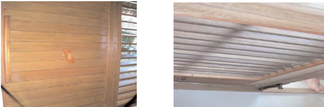
Figure 5.4B Current louver configuration with gaps (right) and well-sealed design (left) (XCO2, 2006)
