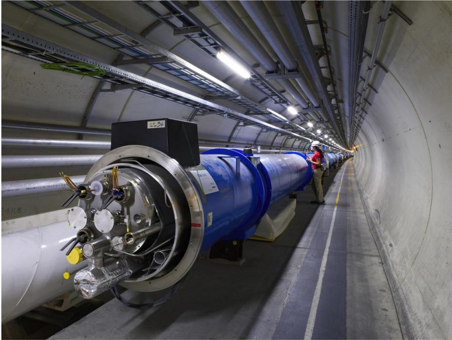
**Figure 2.3:** A LHC dipole magnet under construction.
