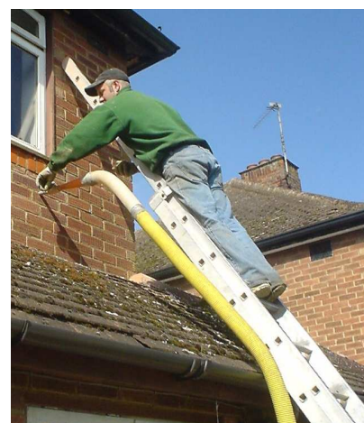
Figure 21.5. Cavity-wall insulation going in.
