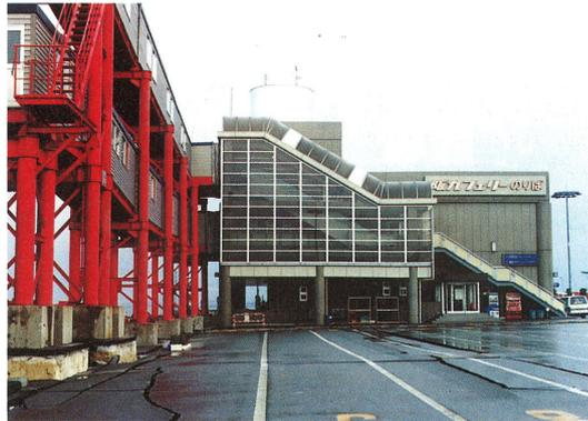
Figure 1.3: Building supported by friction piles showing no apparent differential settlement, Japanese Geotechnical Society (1996)
