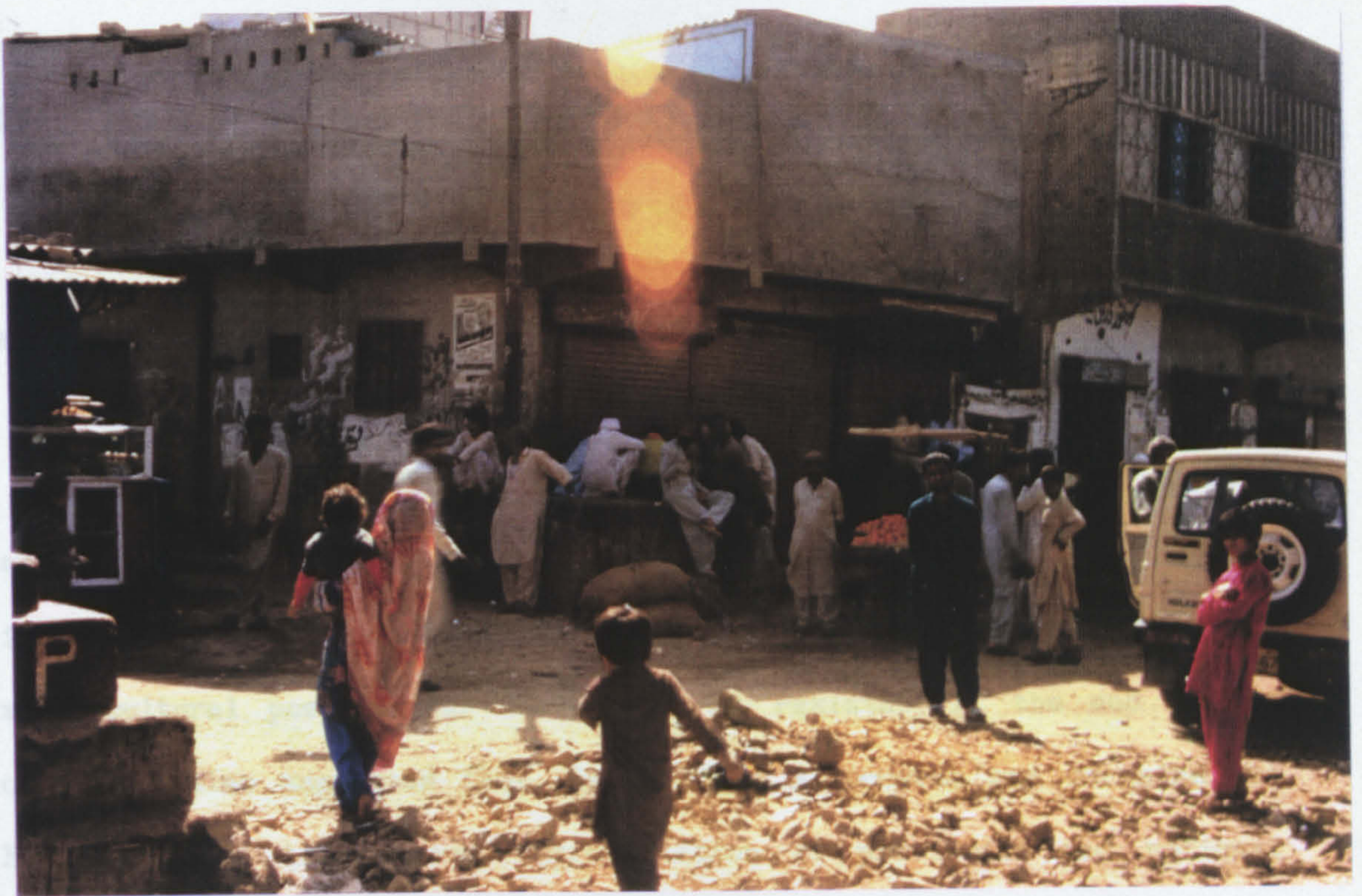
levels, the strata in which the Movement has always been most powerful and has made FIGURE 6.4: Unfinished road, Golimar, Karachi
